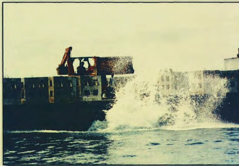
Figure 16 : The anchor-last method applied during the deployment of ARFADs
