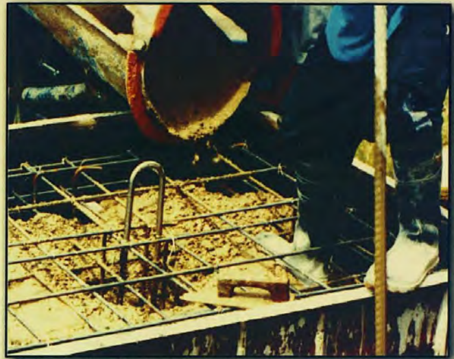
Figure 6 : Details of anchor attachment point (bail). Total length of round stock is approximately 316 cm
