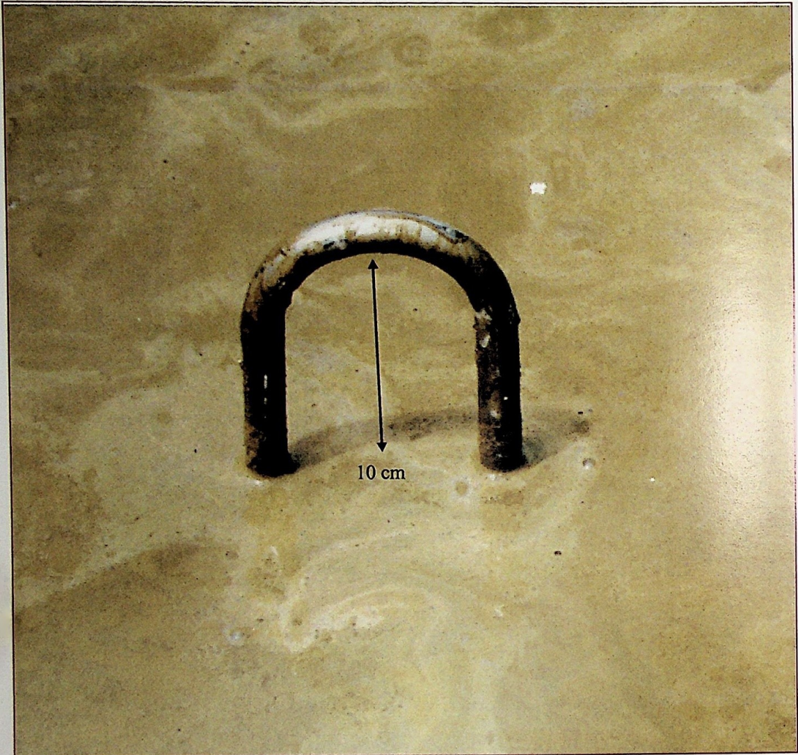
Figure 7 : Anchor attachment point (Bail)
