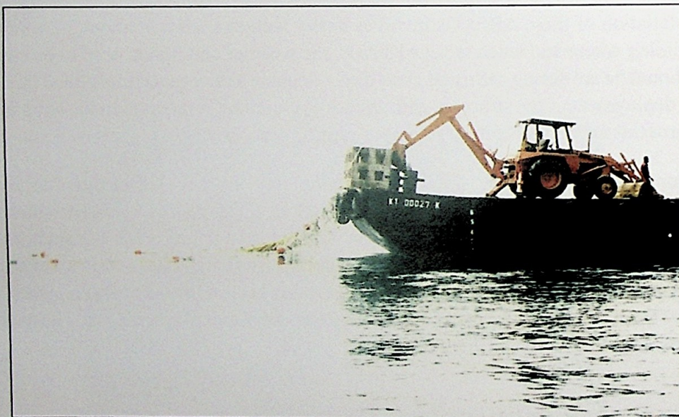
Figure 16 : The anchor-last method applied during the deployment of ARFADs
