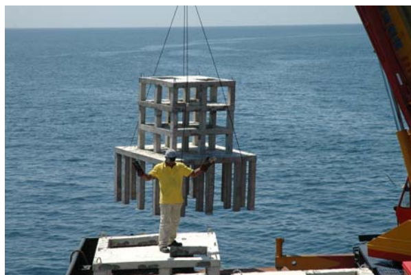
The artificial reef for soft bottom is being deployed in Kedah waters.
