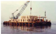
Placement of Artificial Reefs
